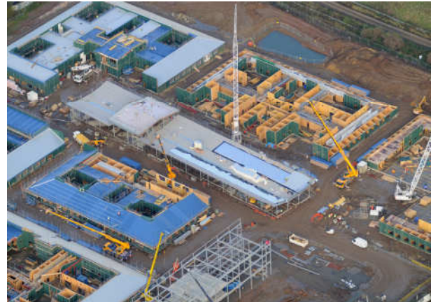
Figure 2. Aerial shot of site
