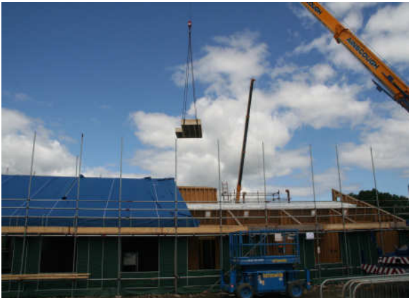
Figure 1. JJI-Joist cassettes being craned
